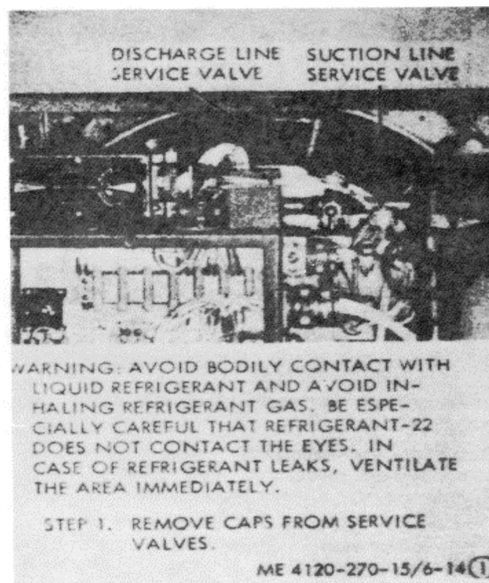
Figure 6-14 (1). Charging refrigerant system.
